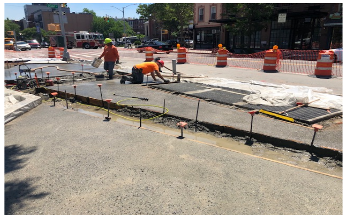
Putnam Plaza: Pigmented and Aggregate Concrete
